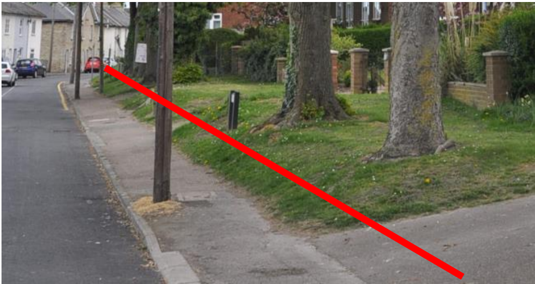
Photo 16 showing area to be widened (approximately) down to c.600- 800mm
